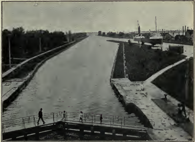
FIG. 256.—The "Soo" Canal. Boats going west pass through the canal on the right; those going east pass through the canal on the left. In the very front of the picture is the gate of a lock.
